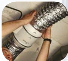
Connect the ducts
