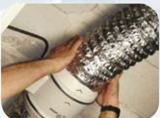
Connect the ducts
