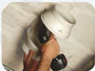
Fix the support bracket
