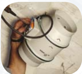
Carry out the wiring connections
