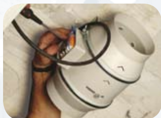
Carry out the wiring connections
