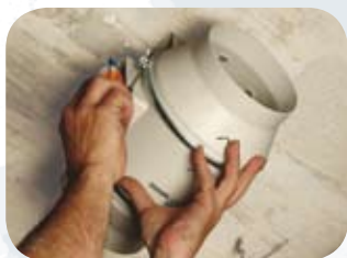
Place the impeller and motor
