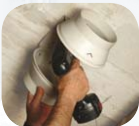
Fix the support bracket
